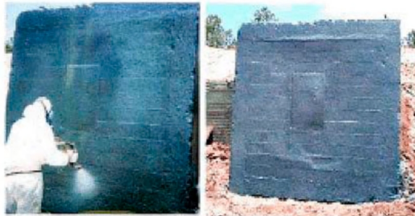
Spraying Polymer
