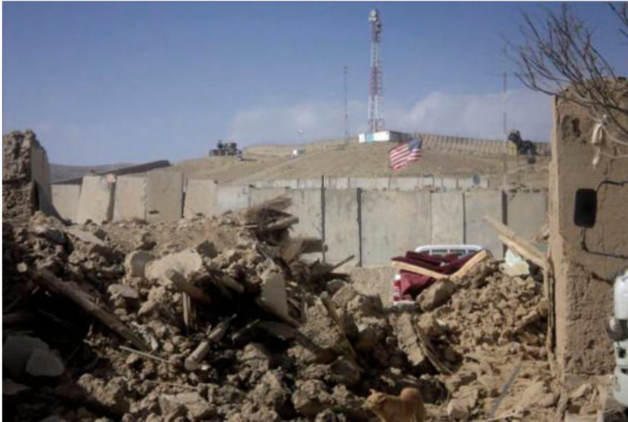
Fig. 1. Aftermath of Truck Bomb attack on US Military Base in Wardak, Afghanistan, 10 th September 2011 [1]
