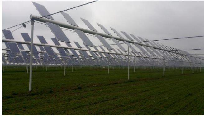
Figure 8. The tensile structures of the Agrovoltaico systems. The source[13]a
