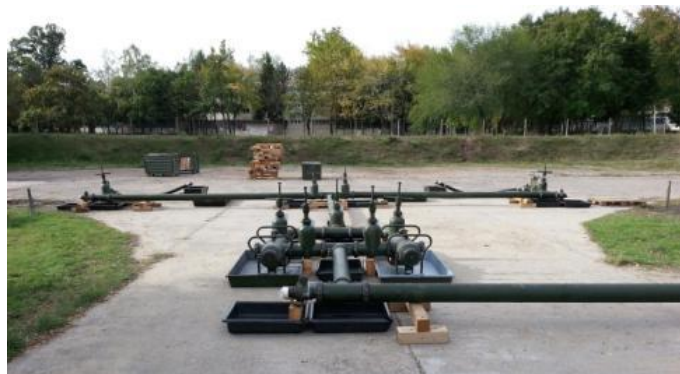
5. Figure. Unloading Section with two ends (Photo made by the author)
