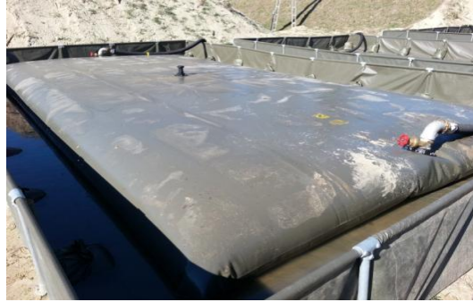
4. Figure. 50 m 3 Flexible Tank in Dyke (Photo made by the author)
