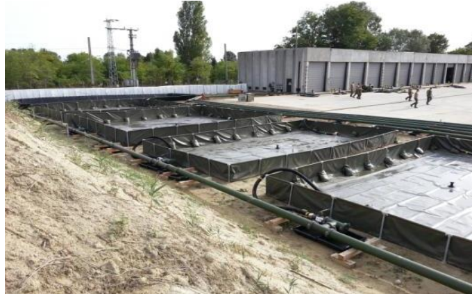
7. Figure. Ground Fuel Section (150 m 3 ) (Photo made by the author)
