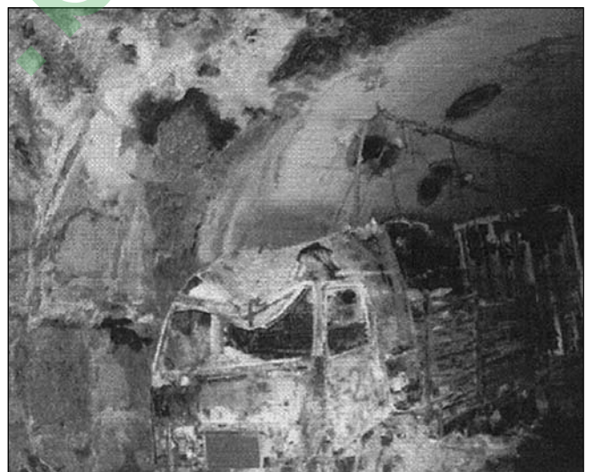
Fig. 4: Damage in the Mont Blanc Tunnel (24. 03. 1999) (Haack, 2002)
