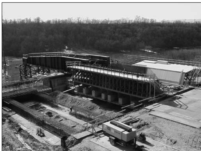
Fig. 2: Constructing deck and launching nose for viaduct S16
