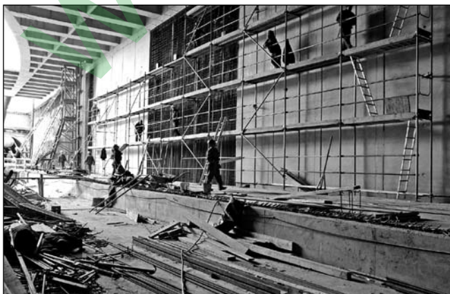
Fig. 6: View of the Tétényi Road station under construction
