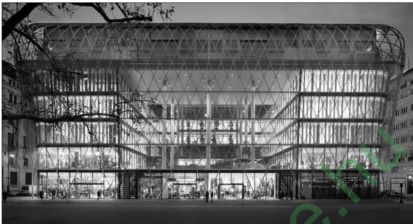
Fig. 10: Vörösmarty Square building in Budapest downtown constructed by Dutch contractors
