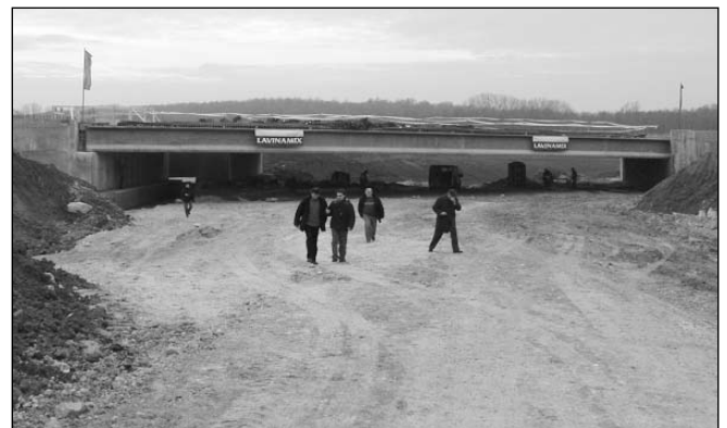
Fig. 8: The superstructure of the Z15 bridge under construction
