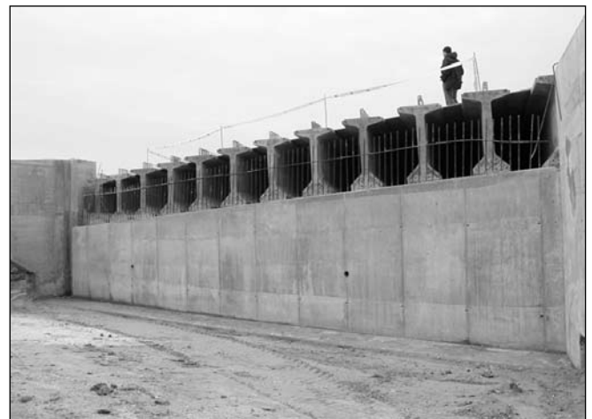
Fig. 9: The abutment and the beam ends
