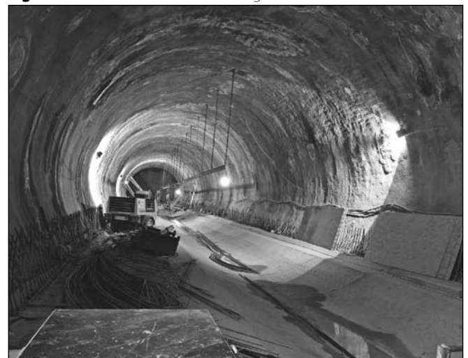
Fig. 2: The the tunnel construction using shotcrete
