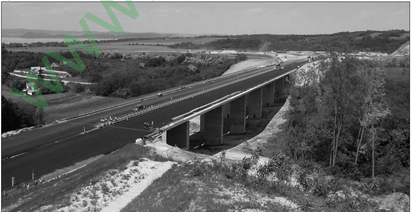
Fig. 1: S16 viaduct – completed
