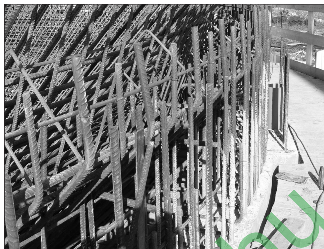
Fig. 13: Reinforcement of the digester under construction in Sopron
