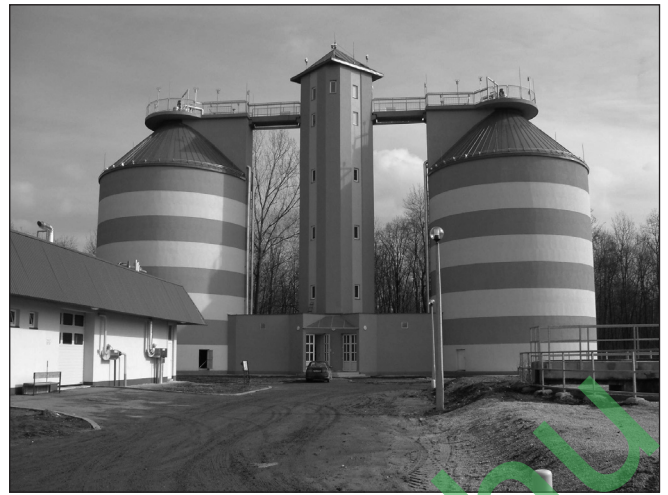
Fig. 3: 2000 m 3 sludge digesters with common staircase in Nyíregyháza
