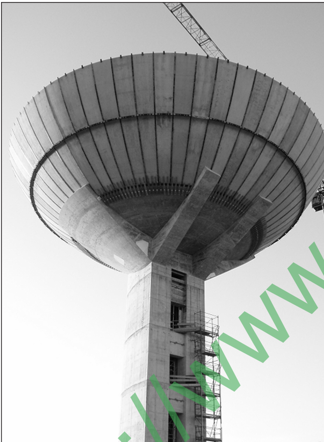
Fig. 2: Construction phase after removing the formwork
