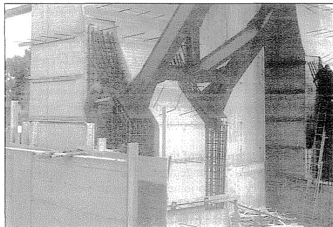
Fig. 5: Bottom of a pier during construction
