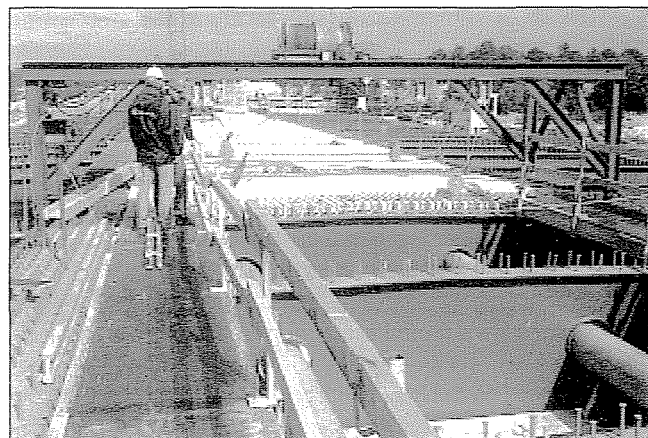
Fig. 7: Installation of a deck slab precast element with a special trolley
