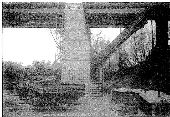
Fig. 4: View of a pier during construction
