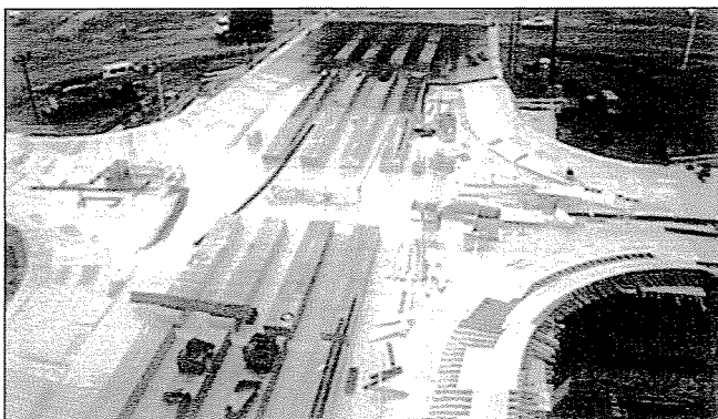
Fig. 9: Crossroads formwork
