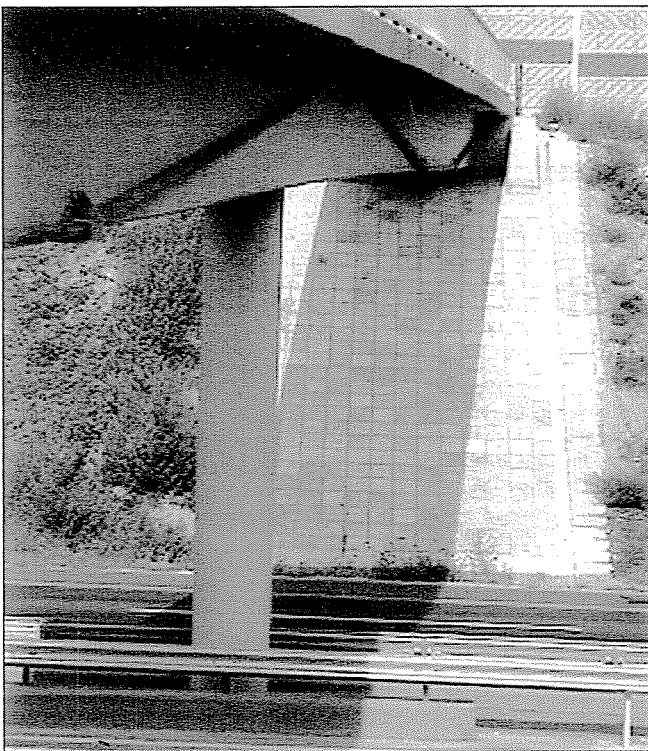
Fig. 7: Bridge at Tetőfedő Street, side view
