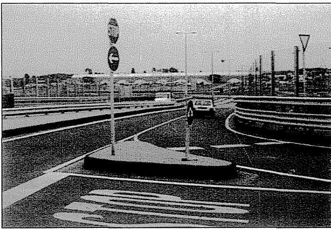
Fig. 16: Road junction on bridge
