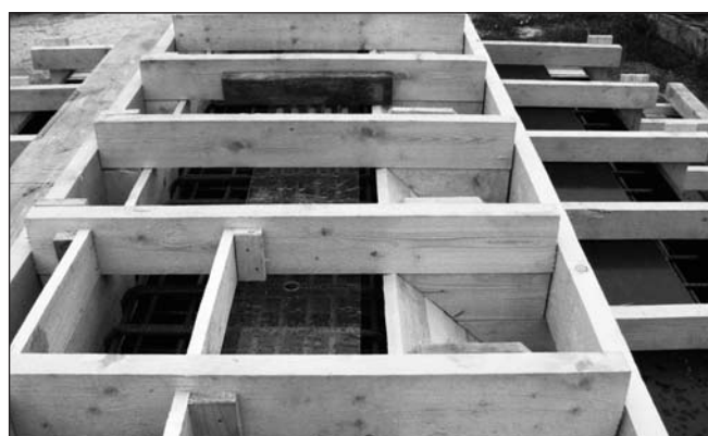
Fig. 7: Asymmetrical trial formwork
