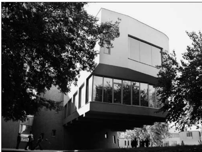
Fig. 3: The cantilever of phase one
