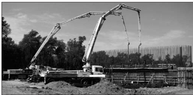
Fig. 4: Tisza Bridge, support No. 5, upgoing wall, Phase I. – concreting works (April 2009)
