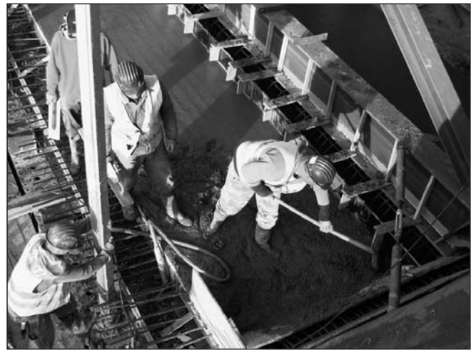
Fig. 10: Concreting of the lower slab (April 2010)
