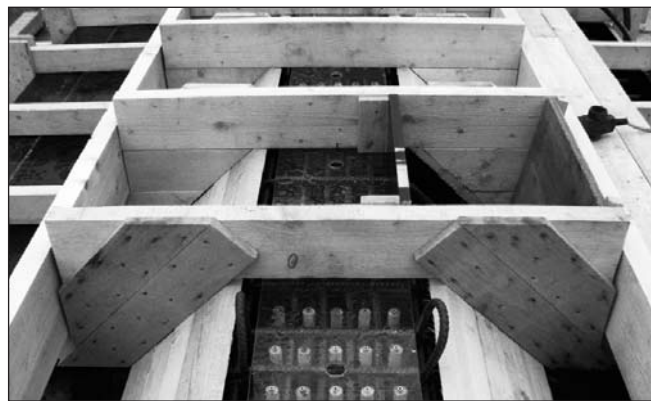
Fig. 6: Symmetrical trial formwork with an opening for concreting
