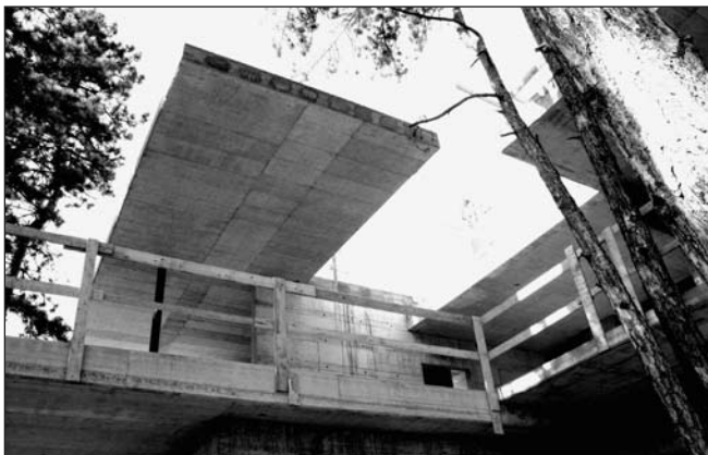
Fig. 1: Bottom view of the cantilever after the formwork had been removed
