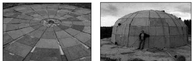
Fig. 30: Transformation of precast divided planar segments into a hemispherical dome (Dallinger and Kollegger, 2009)
