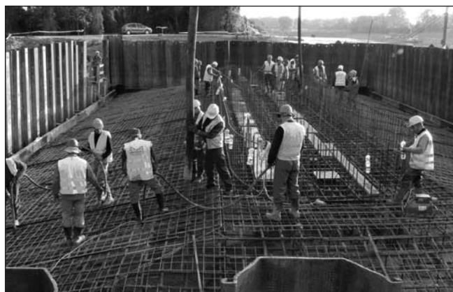
Fig. 3: Concreting of the pile-cap of pier No.6 at Tisza Bridge (May 2009).
