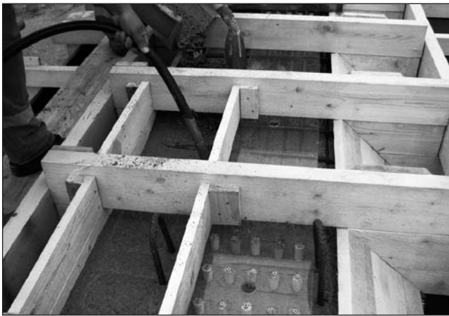
Fig. 8: Asymmetrical trial formwork with a concreting belt
