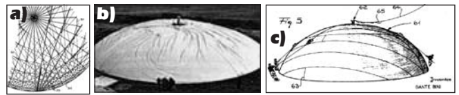
Fig. 29: The binishell system: a) expandable reinforcement (Bini, 1972); b) erection of the dome (Binishell System); c) vibration of concrete after erection (Bini, 1972)
