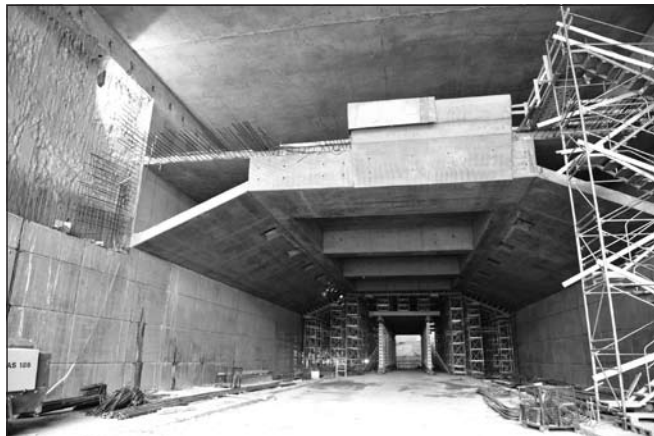
Fig. 6: Completed primary lining of SCL tunnel
