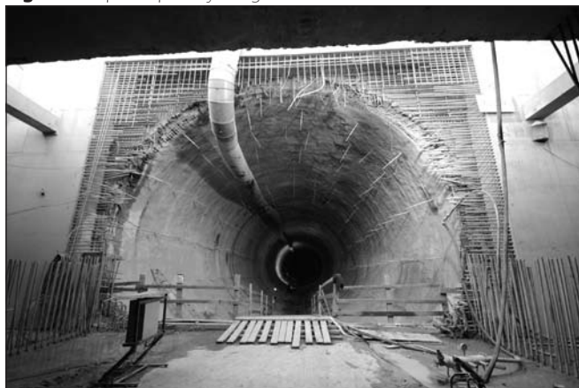
Fig. 6: Completed primary lining of SCL tunnel
