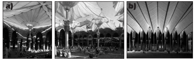
Fig. 26: a) Architectural umbrellas in the courtyard of Mosque in Madinah (Otto, 1995 cited by Walter, 2006), b) Foldable roof in the Rathaus, Vienna (Tillner, 2003; cited by Walter, 2006)
