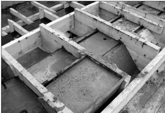
Fig. 9: Symmetrical formwork with an opening for concreting
