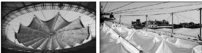
Fig. 24: The retractable part of the Bullfighting Arena roof in Zaragoza (architect: J. Schlaich) (Sobek, 1999; cited by Walter, 2006)
