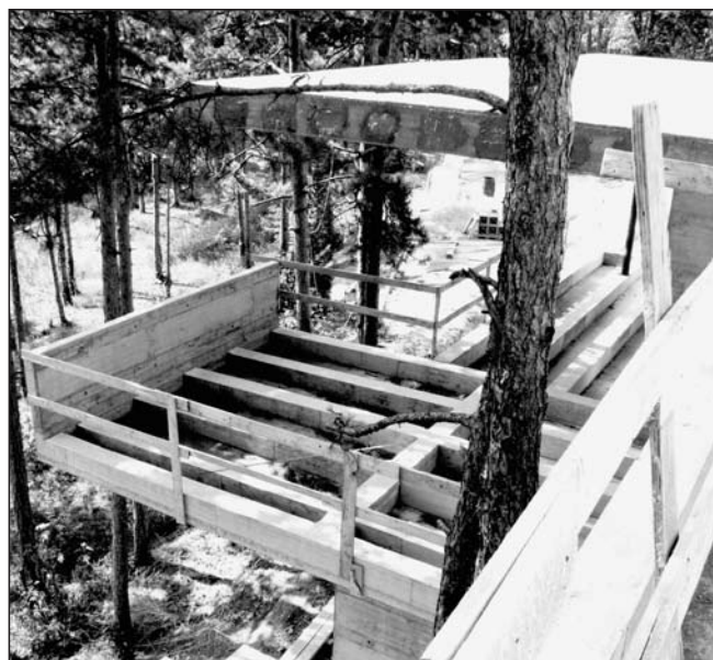
Fig. 4: Side view of the cantilever after the formwork had been removed
