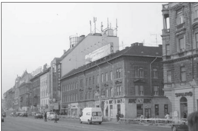
Fig. 6: Buildings affected by ground motions
