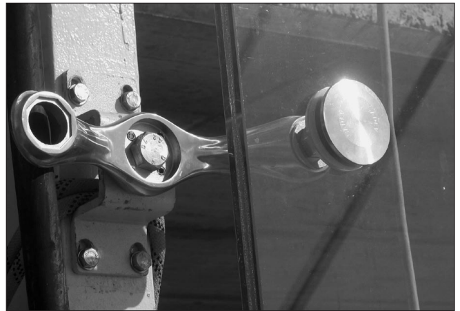
Fig. 11: Point fixing of a glass-wall panel
