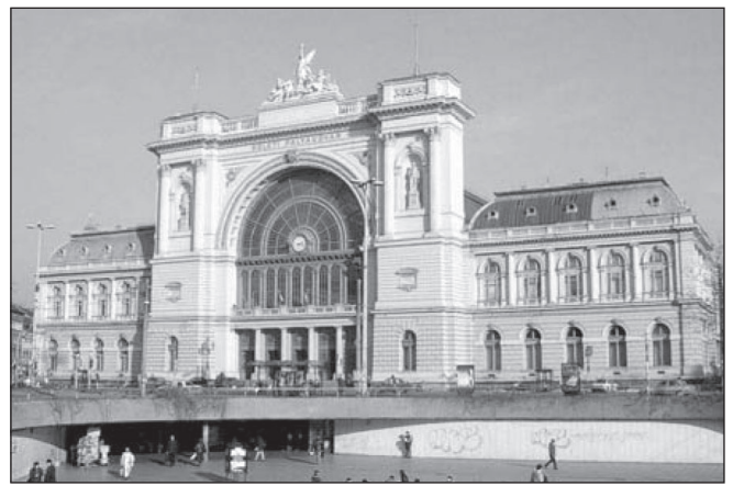
Fig. 7: Main building of the Eastern railway station
