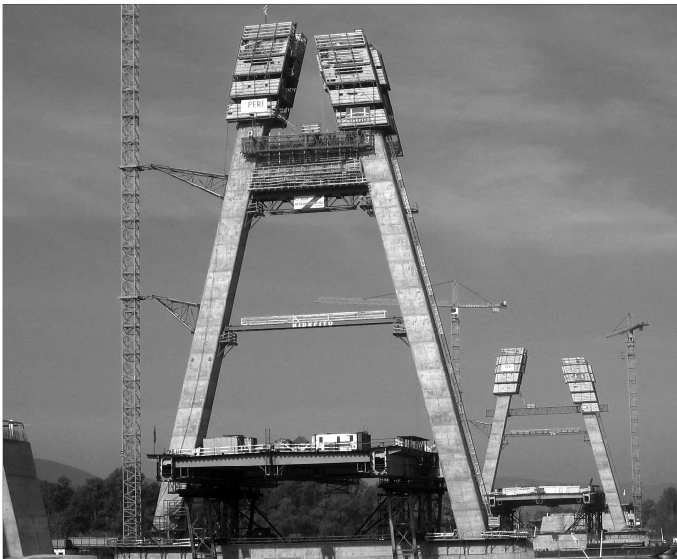
Fig. 7: Pylon legs under construction
