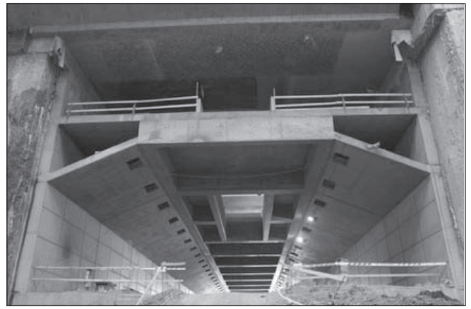
Fig. 4: The station at Kelenföld – passageway under 28 tracks
