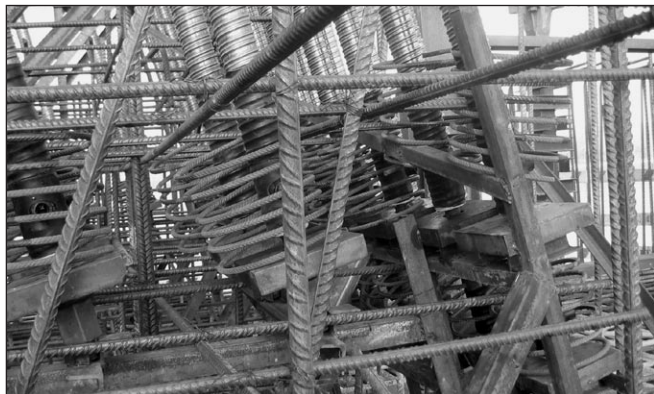
Fig. 5: Anchorage of Ø 40 prestressing bars in a construction joint
