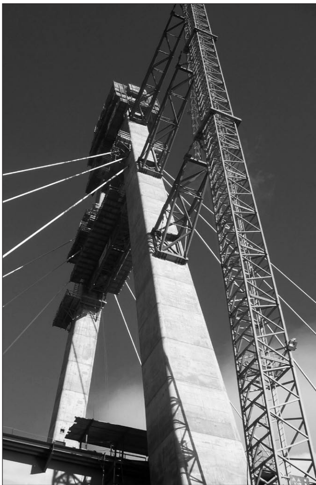
Fig. 8: Tying of a tower crane to the pylon leg
