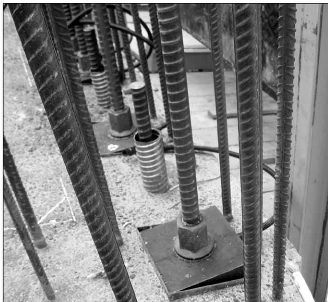
Fig. 5: Anchorage of Ø 40 prestressing bars in a construction joint
