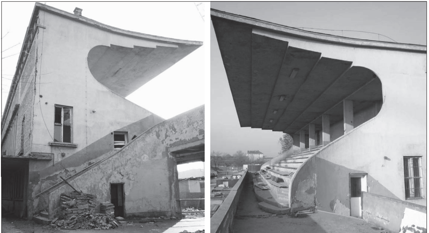
Fig. 1: The Class II Grandstand before renovation
