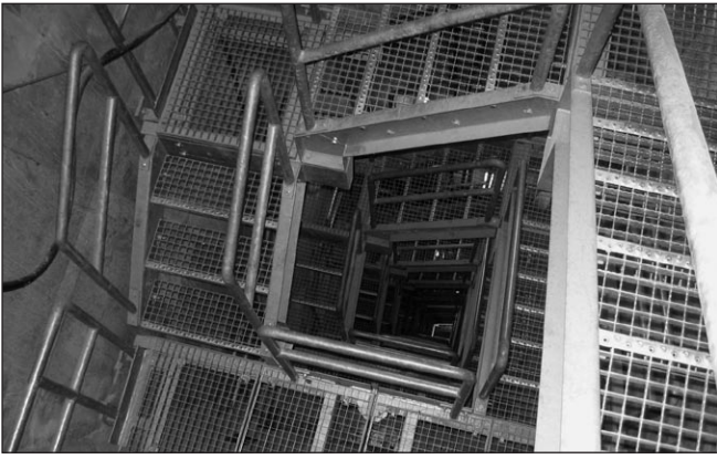
Fig. 12: Inside stairs in the pylon leg
