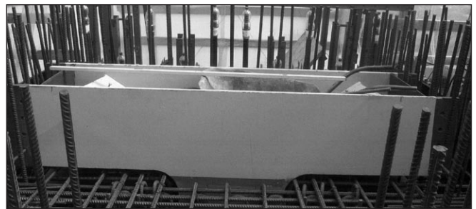
Fig. 6: Steel anchorage device for stay cables
