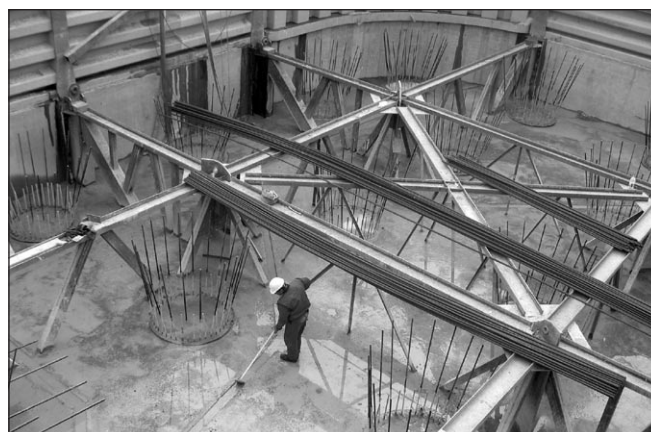
Fig. 3: Pile cap reinforcement above the lower shaft part cast under water
