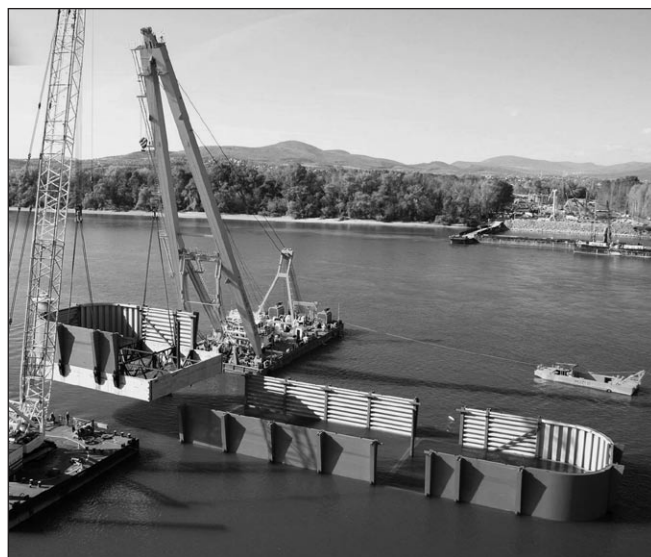
Fig. 2: Positioning of the crib-wall elements
