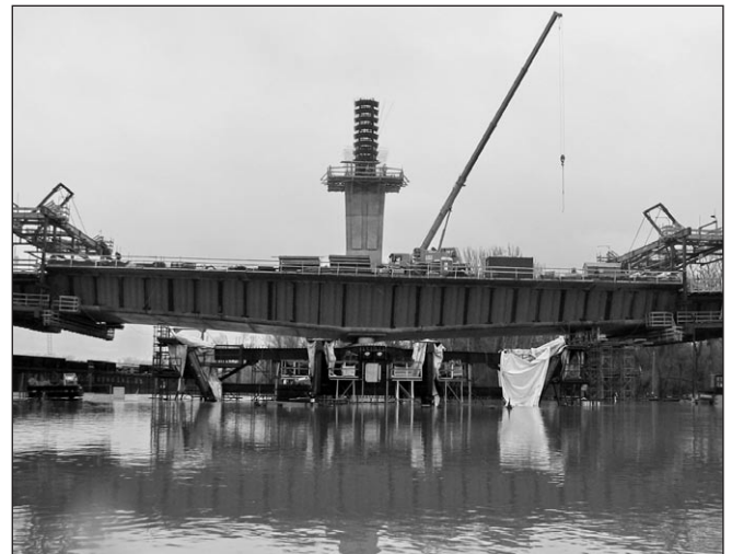
Fig. 5: Building of the bridge with the traveller
