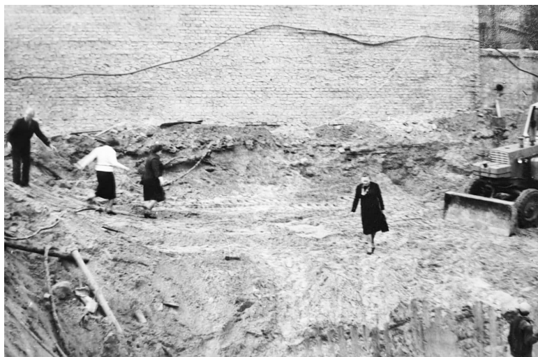
Figure 1. Svetlana Titova (on the right), the director of the Kyiv House of Fashion Design, throws her precious jewelry under the foundation of the new building of the fashion house as it is being laid, 1973. (Private collection of the Kyiv Fashion House designer Lydia Avdeeva, with Lydia Avdeeva's permission)
