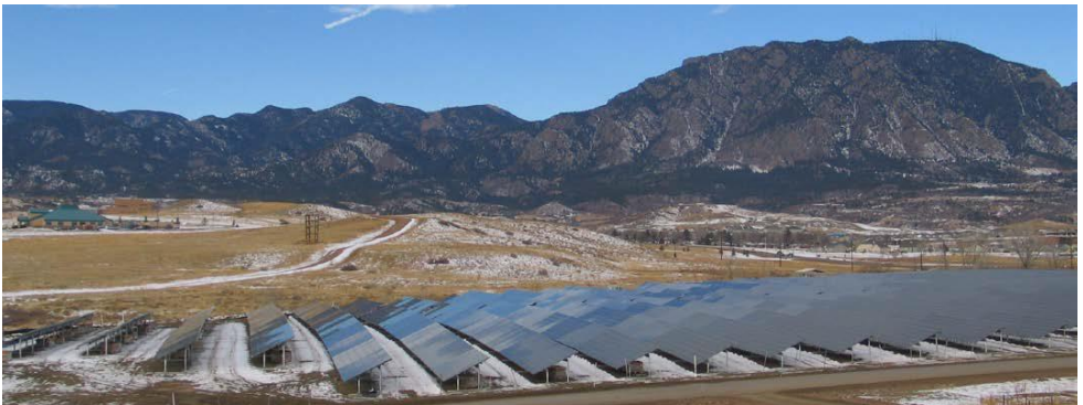
Figure 4: Fort Carson solar array. 11 (9)
