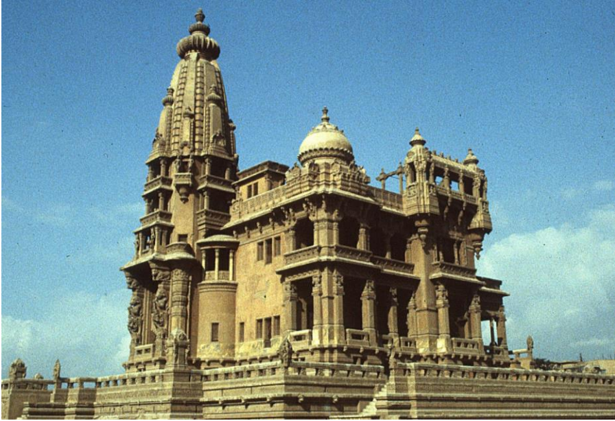
Fig. 10. The Palace of Baron Empain, general view.
