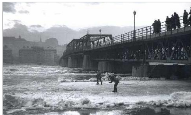
Picture 3. Placing explosives at former Kossuth Bridge, Budapest, 1956 (Source: Kor-képek 1956 - MTI 2006)
