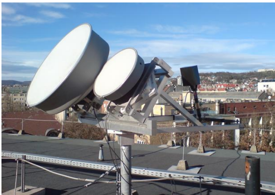
Figure 1. High performance antennas with tracking system
