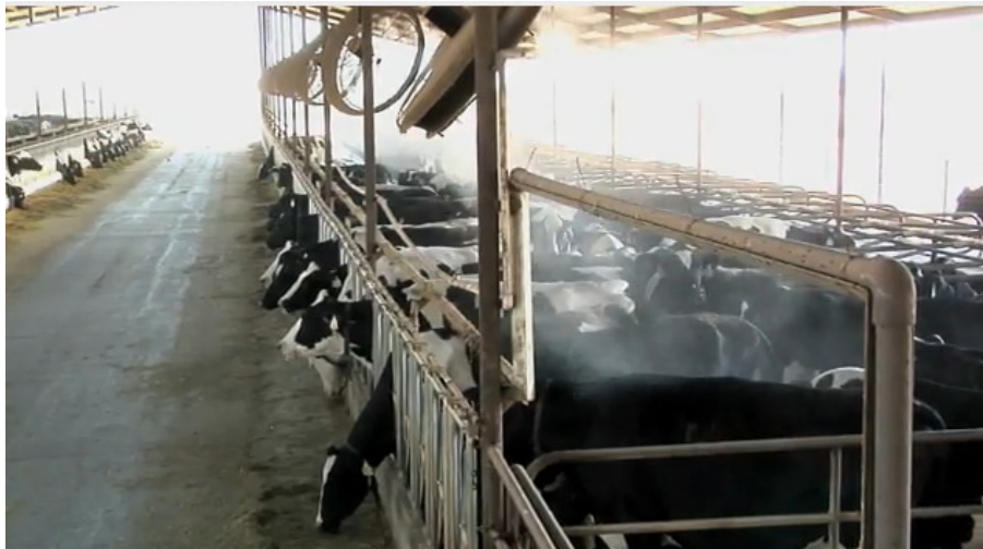
Photograph 12: Naturally ventilated dairy barn with mixing fans and evaporative cooling systems over the feed bunk
