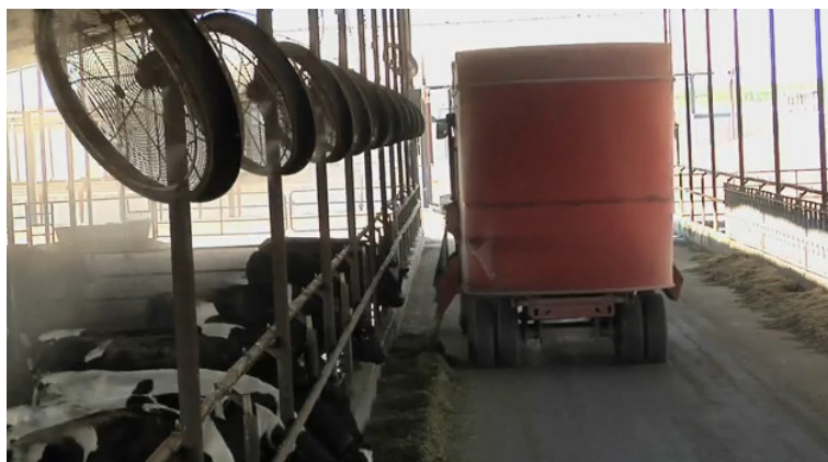
Photograph 11: Sprinkler systems over the feed bunk USA, Minnesota
