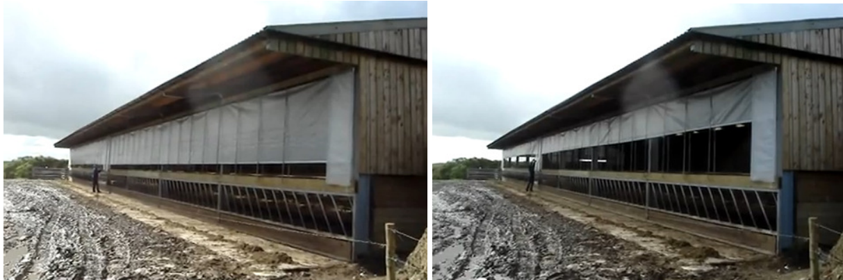
Photograph 2: Opening dairy barn sidewall with manual handle operation
