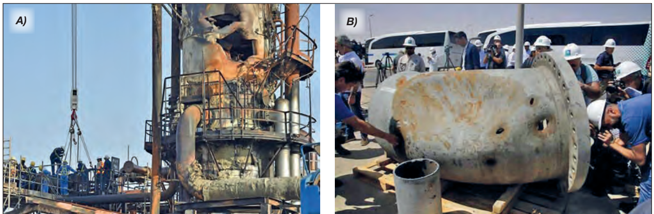
Figure 2. Closer look at the damages
