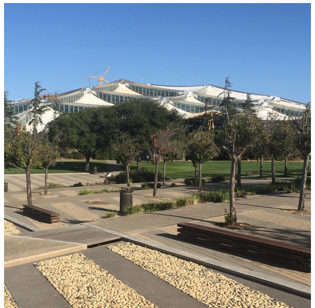
New Google Headquarter, Charleston East, under construction
