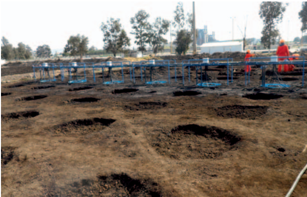
Figure 5. Elektrokinetic remediation in Test site 2 using circular arrangement of electrodes
