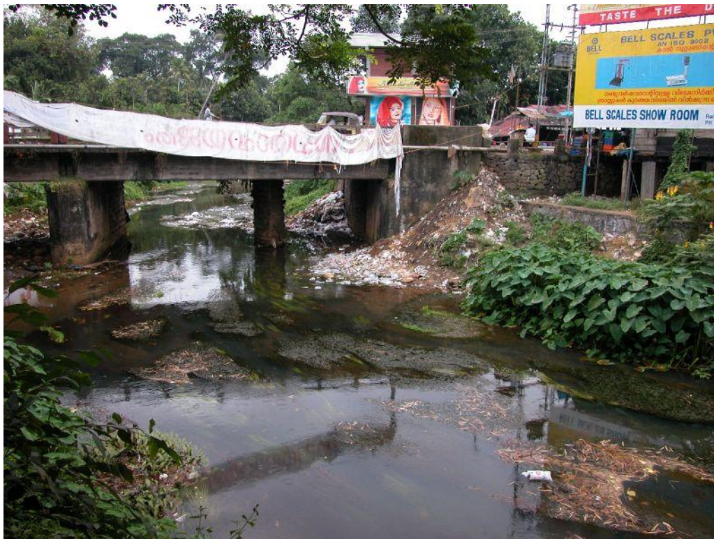
Fig 2: Urban waste disposal site
